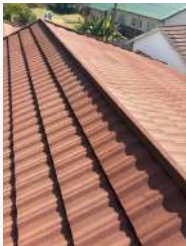
Ref #7 - Roof Exteriors
