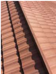
Ref #7 - Roof Exteriors
