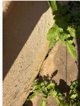
Ref #11.1 - Mold observed on walls
