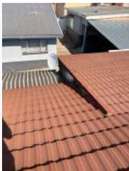
Ref #7 - Roof Exteriors
