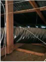
Ref #8 - Roof Cavities
