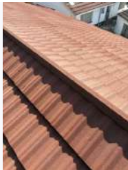
Ref #7 - Roof Exteriors
