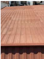
Ref #7 - Roof Exteriors
