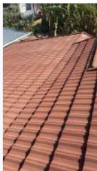
Ref #7 - Roof Exteriors
