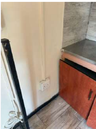
Ref #13.1 - Damaged doors
