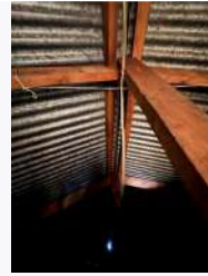
Ref #8 - Roof Cavities
