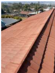
Ref #7 - Roof Exteriors
