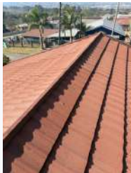
Ref #7 - Roof Exteriors
