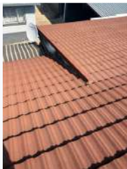
Ref #7 - Roof Exteriors
