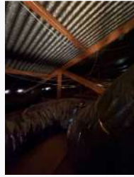
Ref #8 - Roof Cavities
